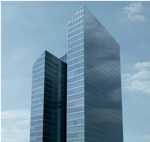
EMS Referenzobjekt: HighLight Munich Business Towers
